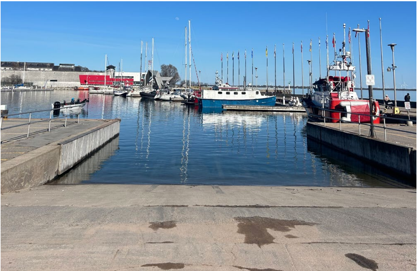
Top left: North ramp. Top right and bottom: South ramp
